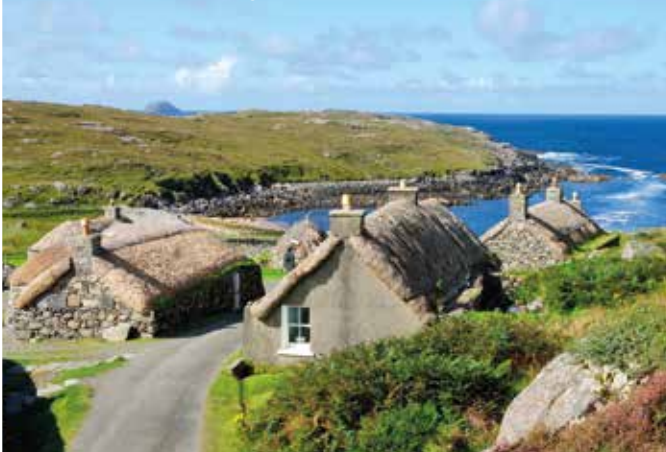
Garrannan Blackhouse Village
